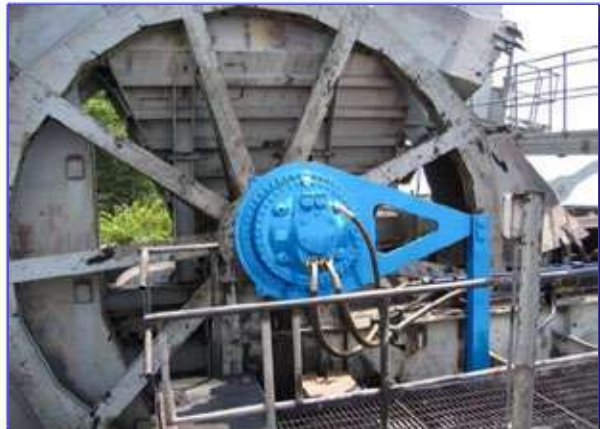
2000 TPH Bucket Wheel Reclaimer Drive Conversion
